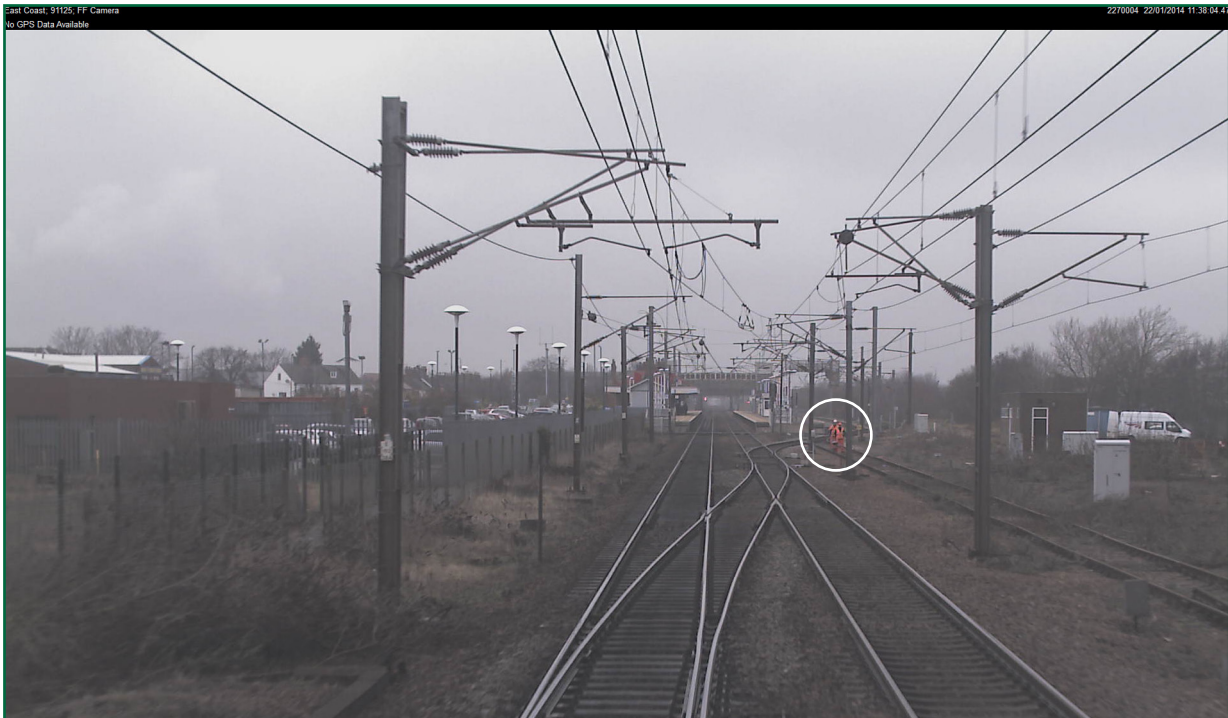
Figure 5: The lookout and tester in the position of safety (image courtesy of East Coast Railways Mainline Company Ltd)
