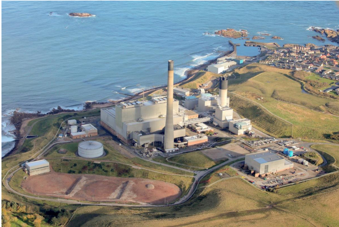
Figure 2-2: Peterhead Power Station
