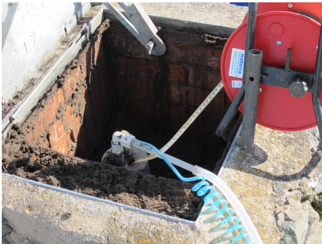
Photo 3 Installed borehole equipment
