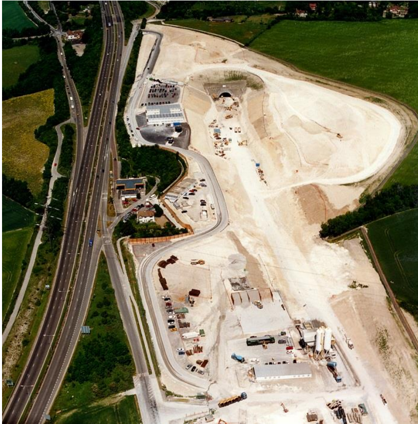
HS1 North Downs Tunnel Portal, Maidstone. Image courtesy of Network Rail
