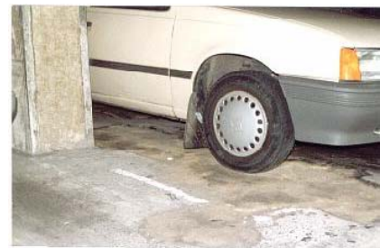
Patch repair of spalled concrete deck
