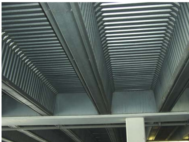
Photograph 23 Typical example of steel deck structure
