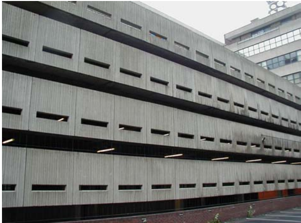
Photograph 21 Typical example of in-situ reinforced concrete frame and slab structure
