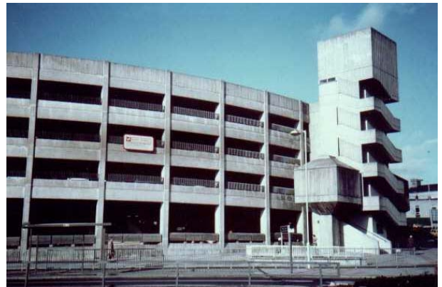
Photograph 22 Typical example of concrete frame structure
