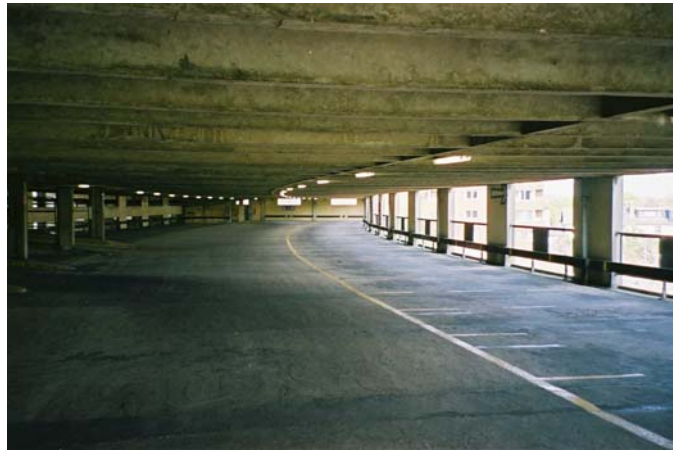
Photograph 1 Wide spans & few supports
