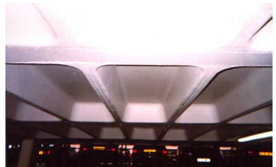
Conductive overlay CP system on an area of soffit.
