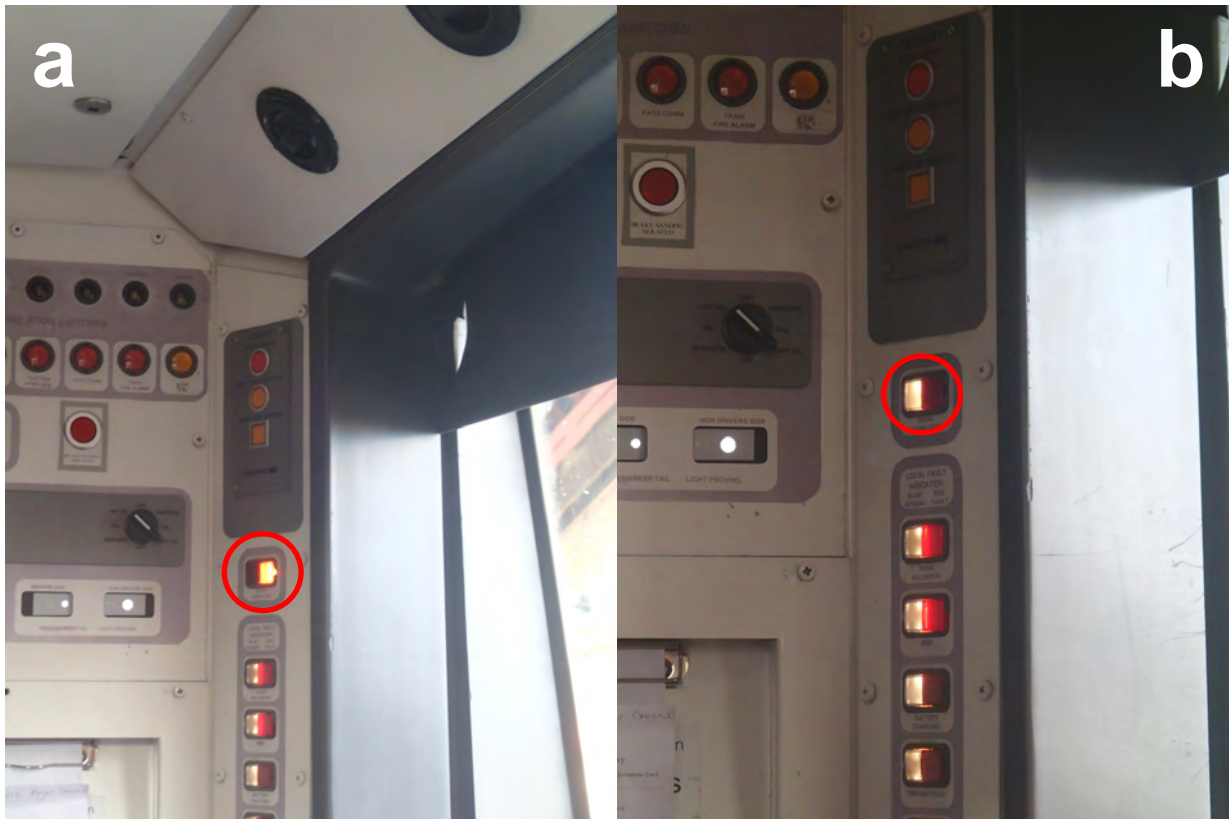
Figure 26: (a) Interlock light providing the driver with indication that the doors are closed and locked and (b) interlock not obtained
