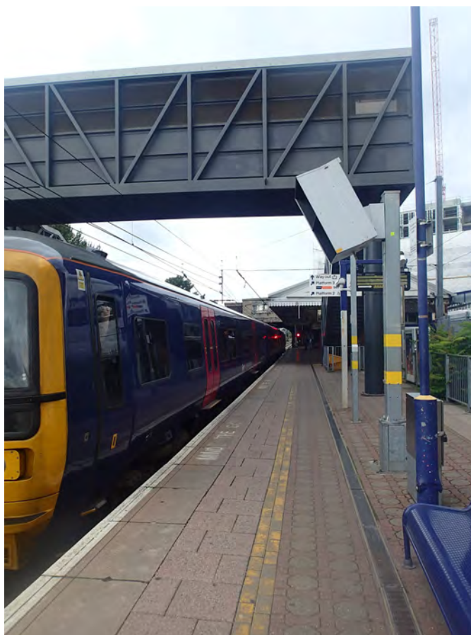
Figure 7: Platform 4 (Up relief line) at Hayes & Harlington
