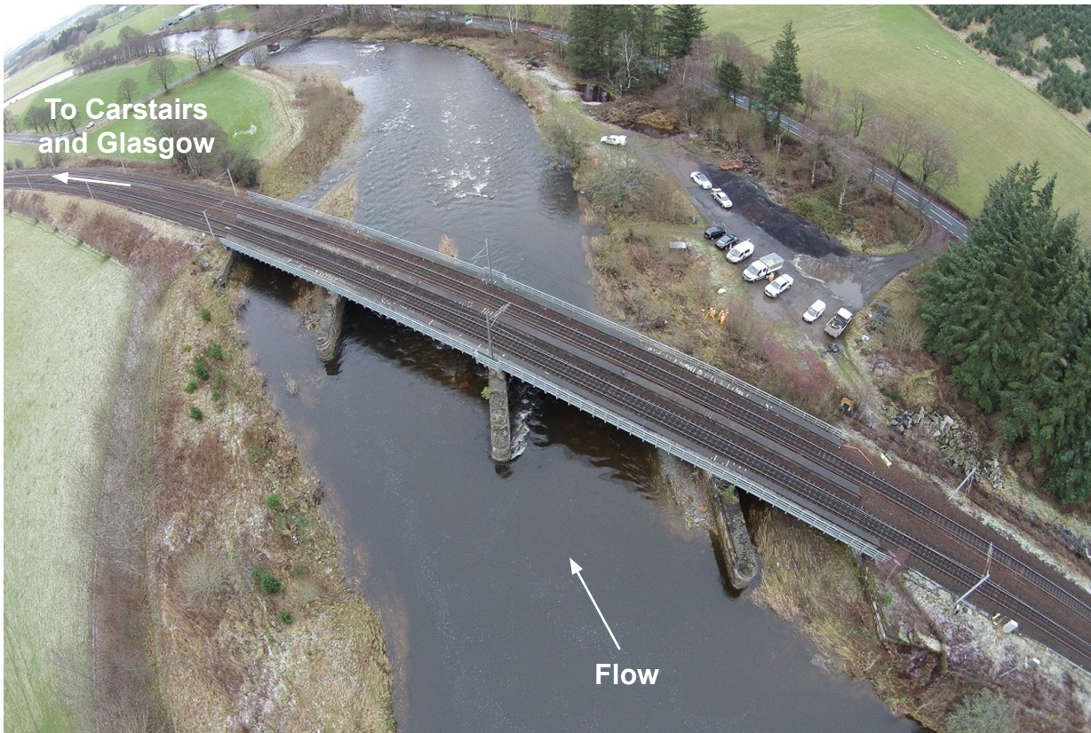
Figure 10: Aerial view on 1 January 2016 (photograph courtesy of Network Rail Air Operations)
