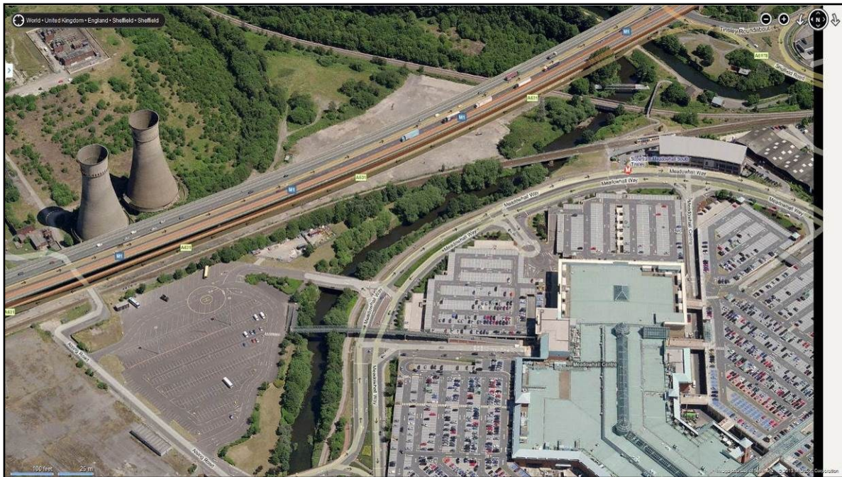
Figure 8.5 – Bird’s eye view of the River Don at Meadowhall Shopping Centre
