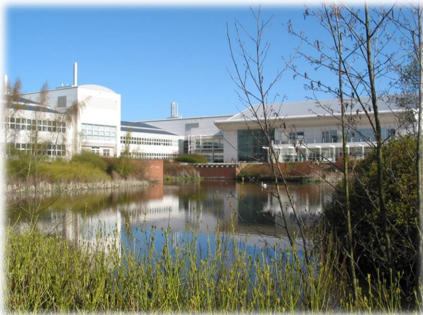
The National Agri-food Innovation Campus, home of the APHA GM Inspectorate.
