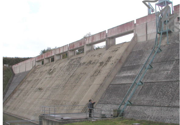
Figure 4.3.7. Eel lift at Bois Joli Dam.
