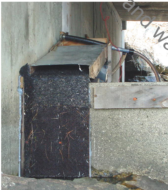
Figure 4.4.10. Vertical substrate board on the west ramp at West Harbor Pond. Photo G. Wippelhauser
