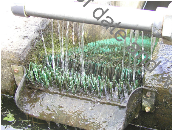
Figure 4.3.9 Sprinkler water inlet at top of elver pass, Bois Joli
