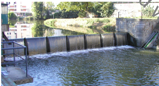
Figure 4.3.20. Eel pass at Rennes Weir
