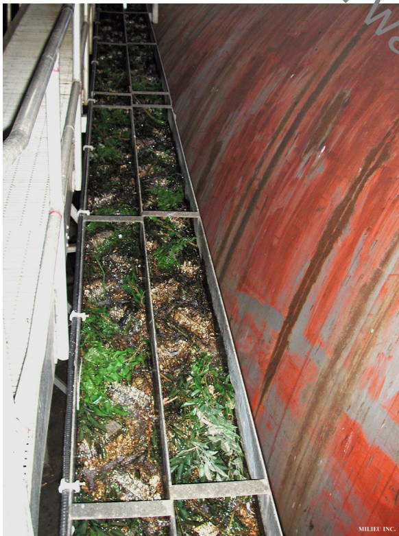
Figure 4.4.2. Details of the double channel pass at Moses-Saunders Dam. Photo D. Desrochers
