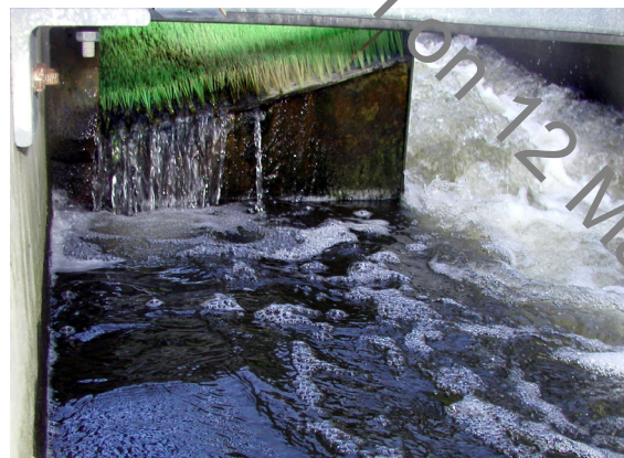
Figure 4.2.14 Downstream end of Abingdon eel pass in June 2003, showing tail-water level well below the bottom of the pass
