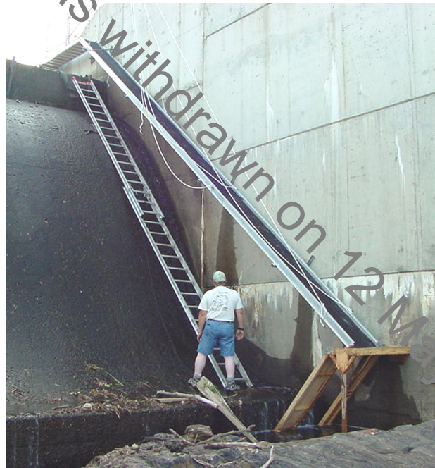
Figure 4.4.9. Pass at Benton Fall Dam. Note layout to ensure entrances to pass are close to the dam face. Photo G Wippelhauser
