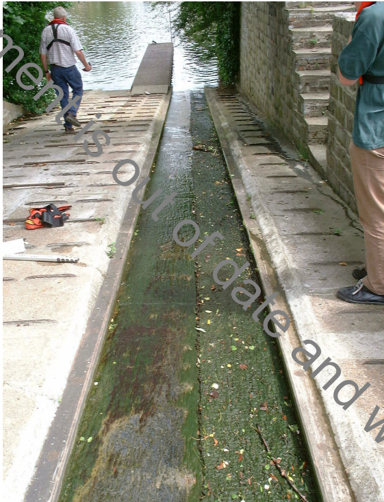
Figure 4.2.11 Canoe ramp at Sunbury lock showing Enkamat elver substrate on right-hand side.
