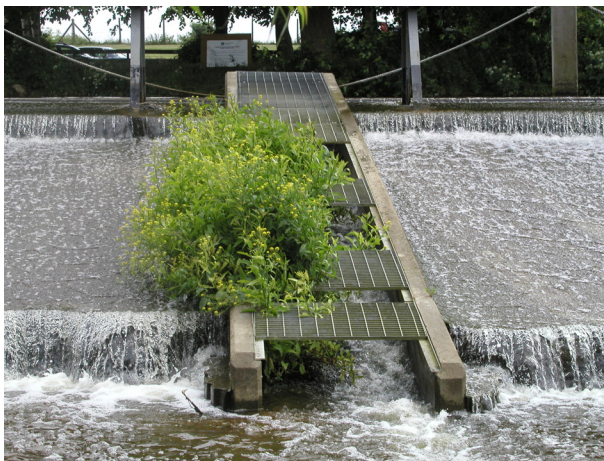
Figure 4.2.12. Sunbury Weir elver pass
