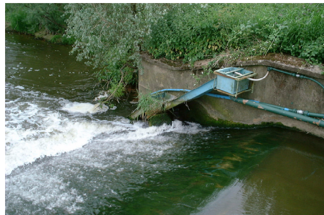
Figure 4.2.7 Right-bank eel pass at Strensham Weir. It has been severely damaged during a flood by a log that is still jammed beneath the resting pool.
