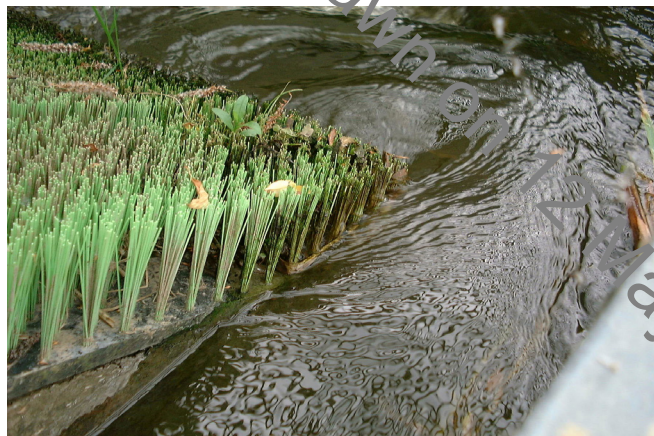
Figure 4.2.10 The top end of the bristle substrate mat pass on the left bank at Evesham Weir. Note how the flow entering the baffle part of the pass cut across the upstream end of the substrate mat
