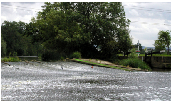
Figure 4.2.8. General view of Chadbury Weir showing left-bank eel pass
