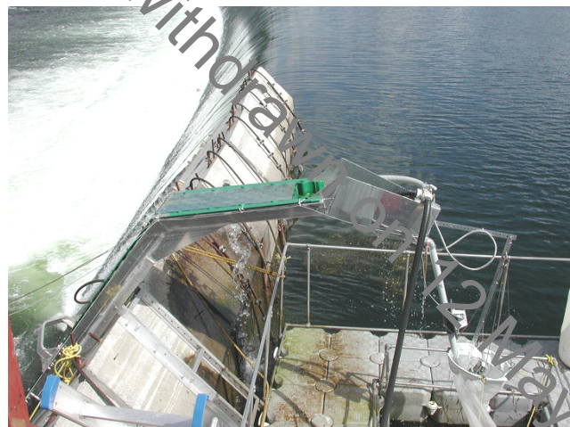
Figure 4.4.4. View of Chambly Dam eel pass from above. Note breakwater blocks on dam crest, covers over the channel containing "Eel-ladder" substrate, and electronic counting device on the pipe carrying the eels from the top of the pass to the keep net with its flotation collar. Photo D. Desrochers
