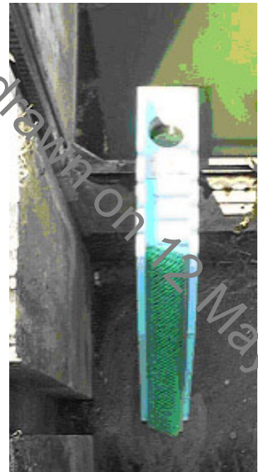
Figure 4.3.24. “Fish-Pass” prefabricated sluice gate pass
