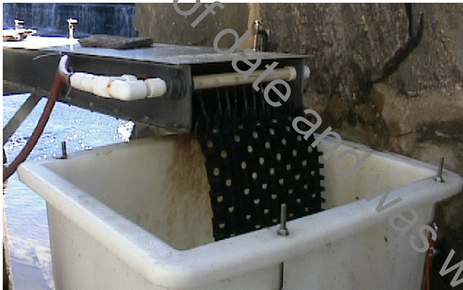
Figure 4.4.14. Akwadrain substrate extending beyond top of ramp at Greeneville Dam eel pass. Photo A Haro
