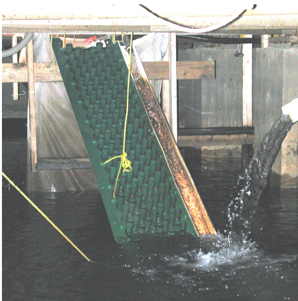
Figure 4.4.5. Earlier eel pass-trap at Beauharnois, using “Eel-ladder” substrate. Note attraction flow. Photo D. Desrochers
