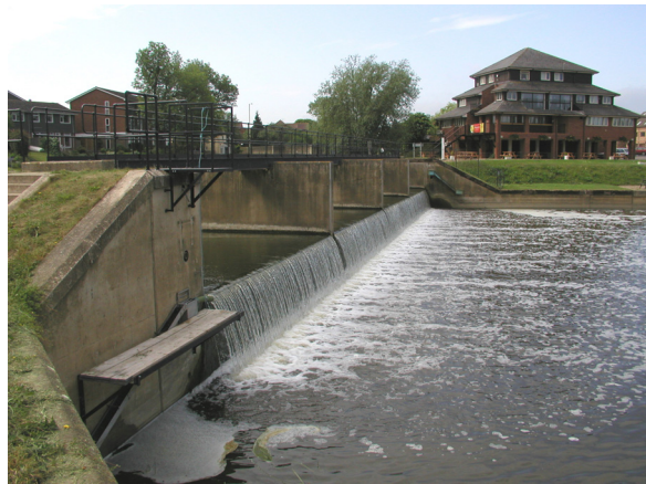
Figure 4.2.3 Elver passes at Stanchard Pit Weir
