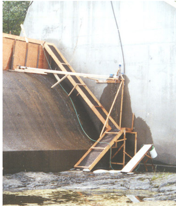
Figure 4.4.8 Pass at Fort Halifax Dam. A “portable passage” ramp is being deployed alongside. Note layout to ensure that entrance to pass is close to the face of the dam. Photo G Wippelhauser
