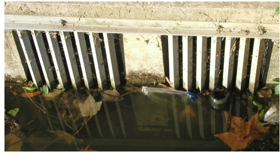
Figure 4.3.22. Trash screen at the upstream end of eel pass at Rennes Weir
