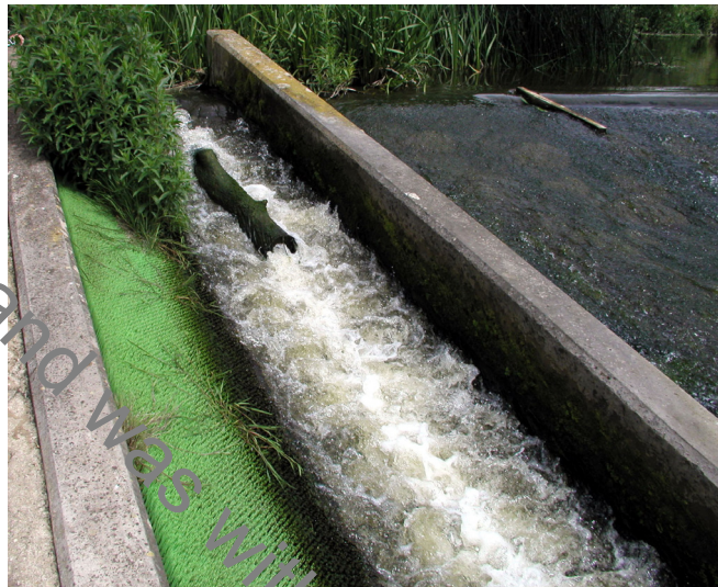
Figure 4.2.9 Bristle substrate and baffle fish pass at Chadbury Weir
