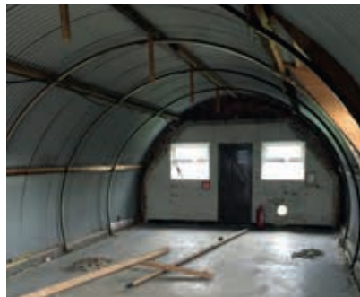
A stripped out Nissen hut before refurbishment © Landmarc Support Services
