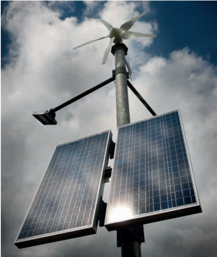
LED site lighting, powered by wind and solar panels © AWE
