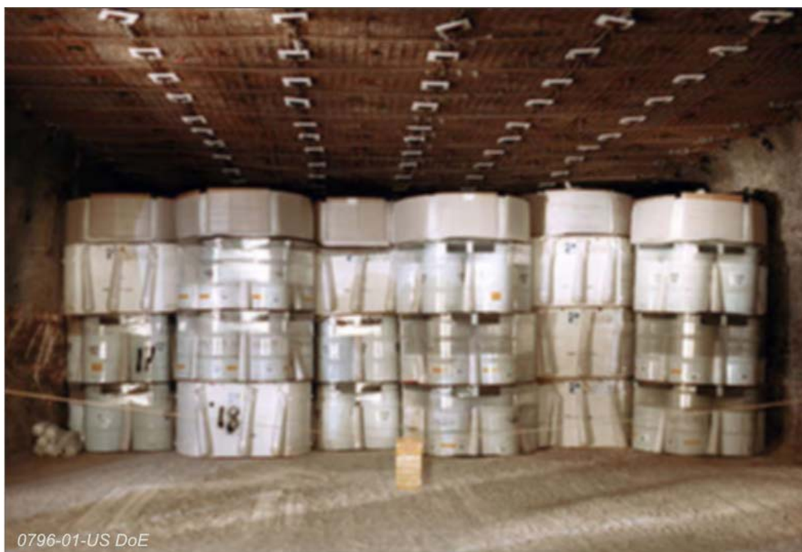
Waste Isolation Pilot Plant (USA) Evaporite rocks (salt deposits) provide a dry environment and are in use in the USA and Germany
