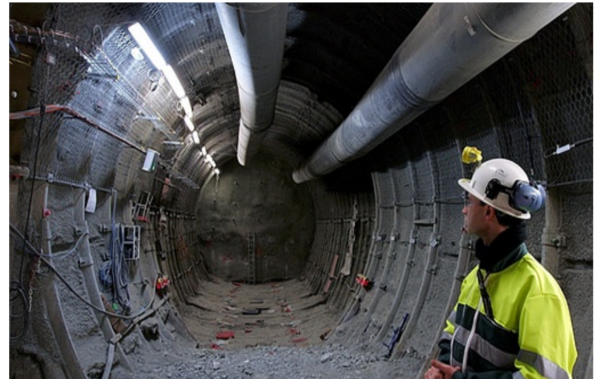
ANDRA underground test and research site (Bure, France) Lower strength sedimentary rocks, such as clays and mudrocks are proposed as host rocks in France and Switzerland
