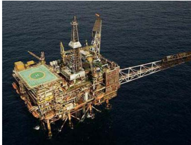
Figure 02 – Fixed Platform with modular drill installed.
