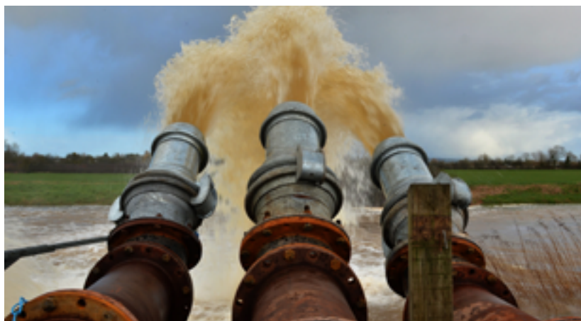
Royal marines pump floodwater into the River Parrett at the Saltmoor Pumping Station near Burrowbridge in Somerset.
