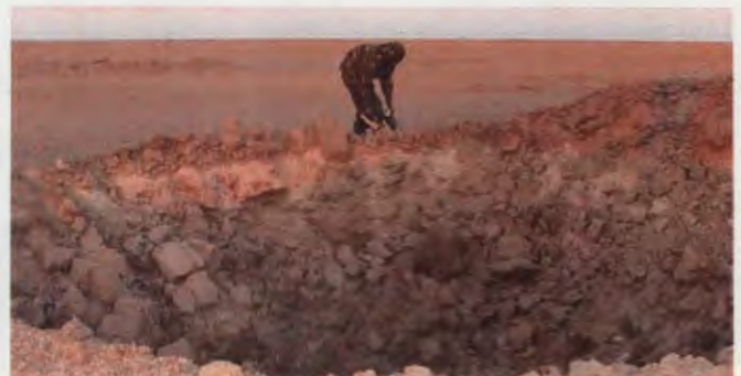
Fig. 3: CBRN Team Red operator conducts post-demolition site survey in order to ensure that no contamination remains on the site.
