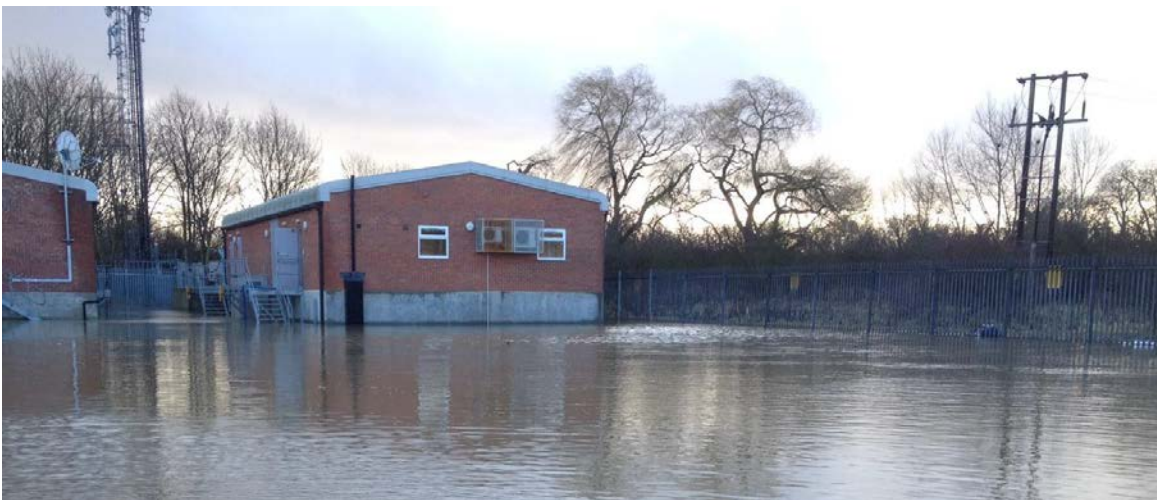
Bushey Mill Grid Substation (February 2014) showing elevated Switchhouse and control rooms
