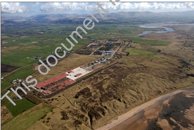
Photograph of the LLWR taken from the north west, courtesy of LLW Repository Ltd
