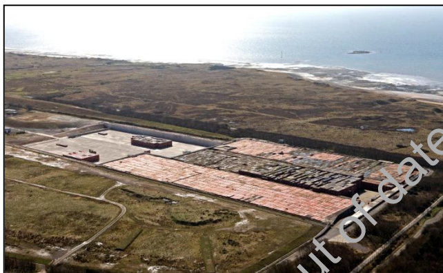
Photograph of the northern end of the LLWR taken from the north east, courtesy of LLW Repository Ltd
