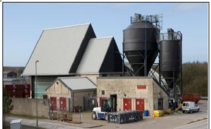
The LLWR Grouting Facility, courtesy of LLW Repository Ltd
