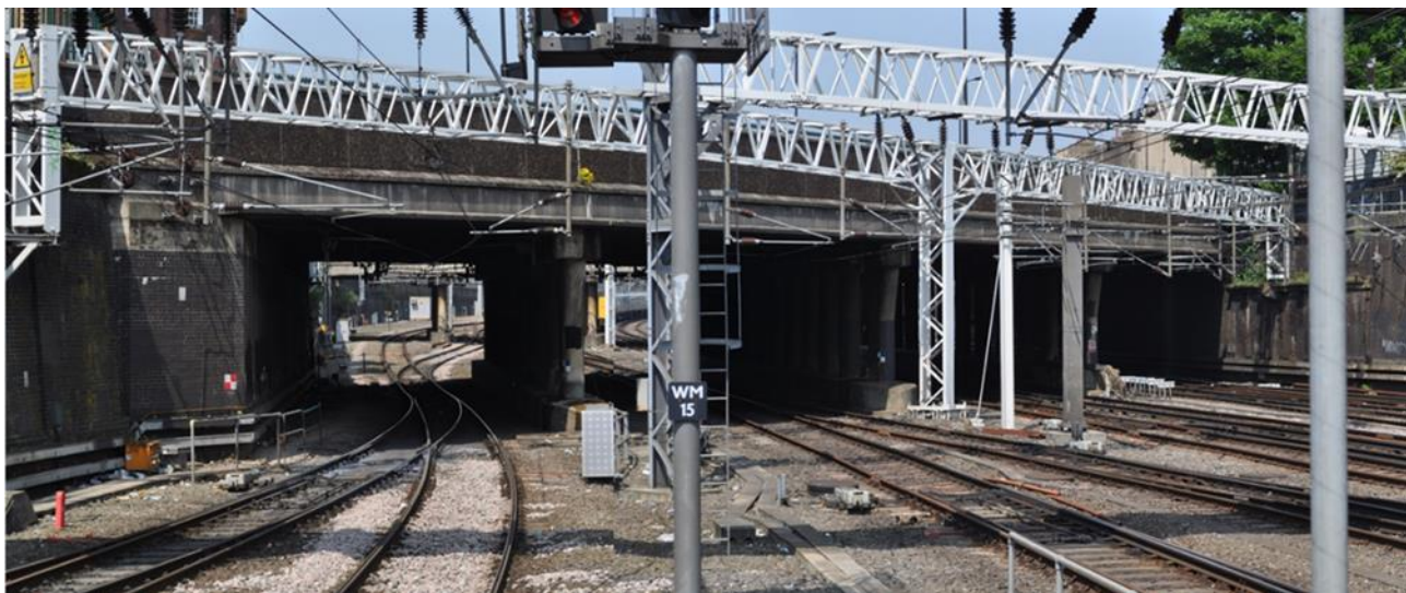
Figure 22: Picture of the existing HRB over NR
