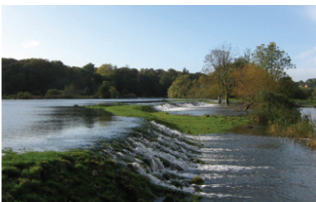
Overtopping at Postwick Marshes, River Yare
