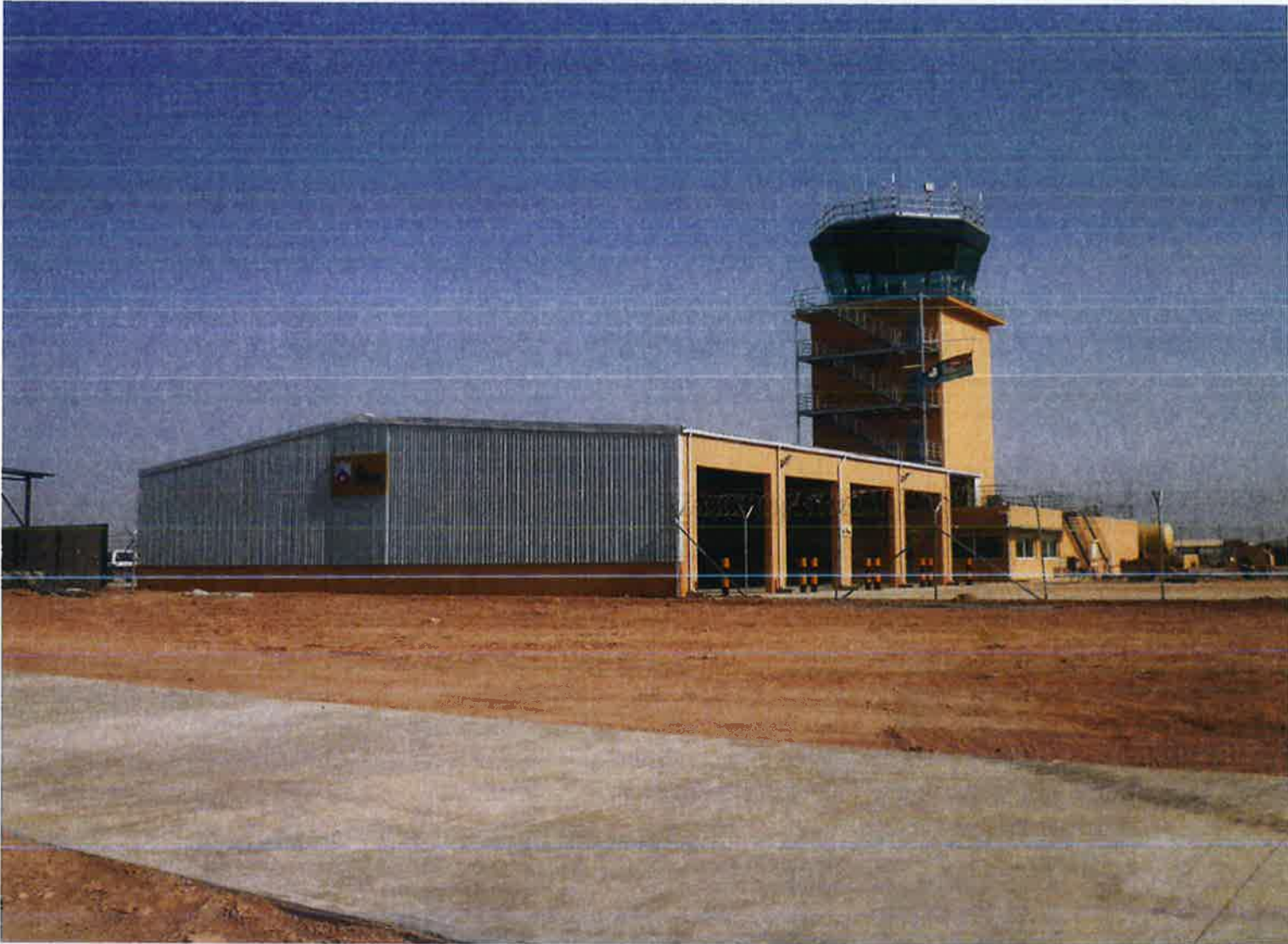
Figure 4-4-6. The new air traffic control tower
