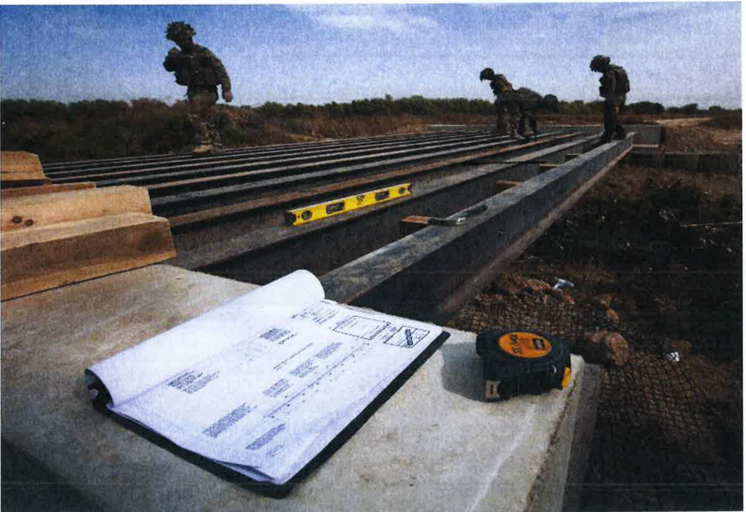
Figure 3-7-6. Improvised sustainable bridging.
