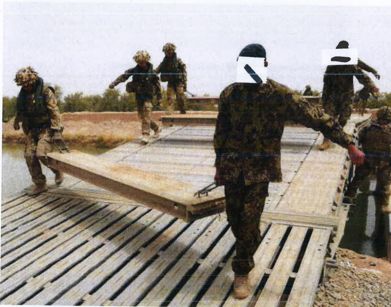
Figure 3-7-9 Bridge deck stripping with ANSF Engineers
