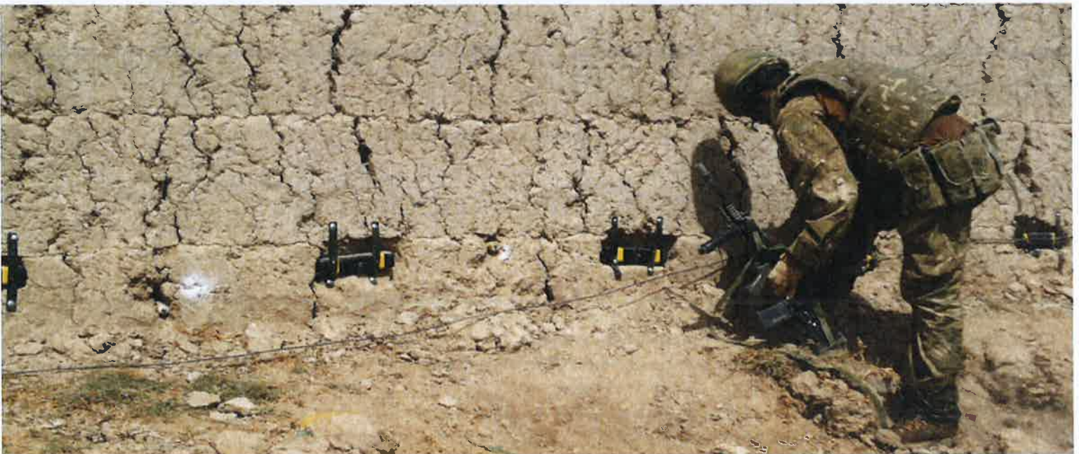
Figure 3-7-1. Final preparations for compound wall demolition
