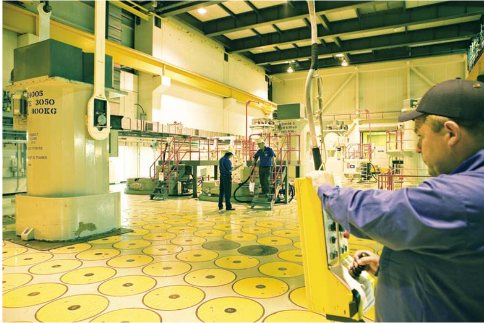
Figure 26: Vitrified Product Store (VPS) at Sellafield
