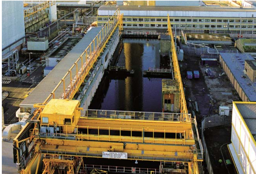
Figure 29: Pile Fuel Storage Pond (PFSP) at Sellafield
