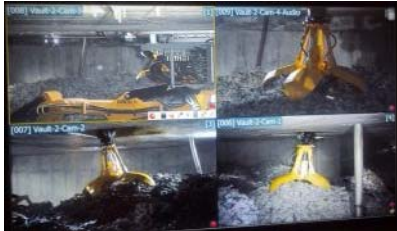
Figure 34: Video feeds from inside the Fuel Element Debris (FED) vault at Berkeley
