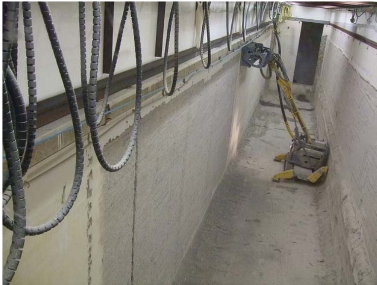
Figure 41: Scabbling of the pond walls at Trawsfynydd
