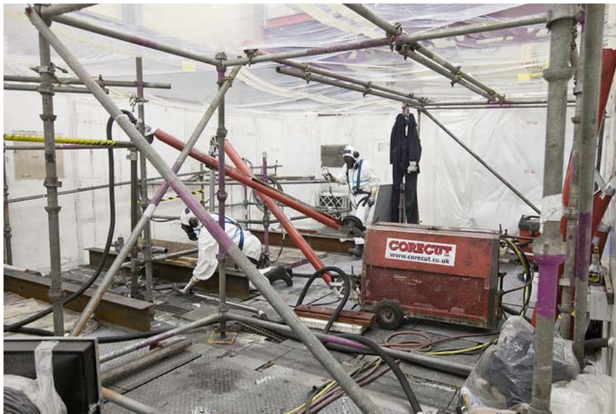
Figure 40: Decommissioning of Dounreay Material Test Reactor (DMTR)
