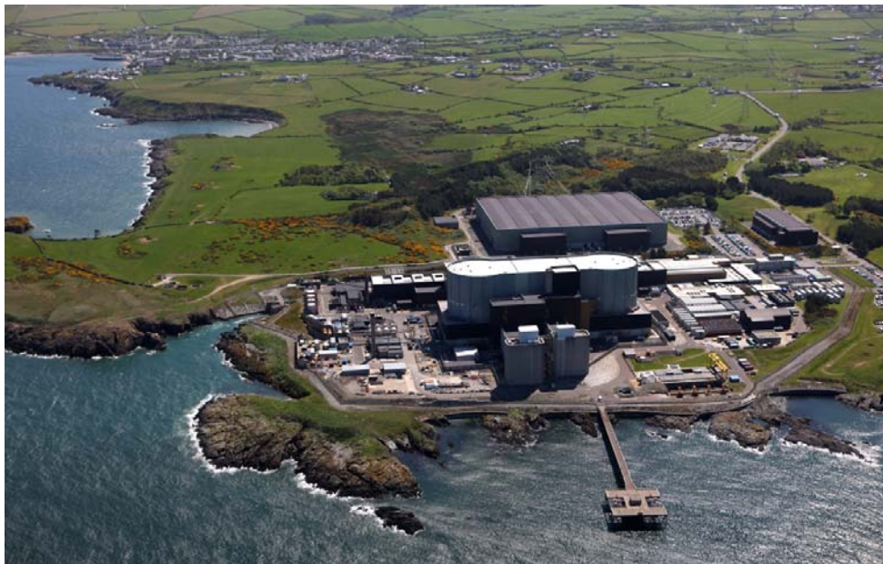
Figure 7: Aerial view of the Wylfa Magnox power station
