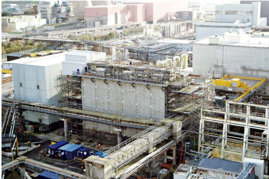
Figure 31: Pile Fuel Cladding Silo (PFCS) at Sellafield
