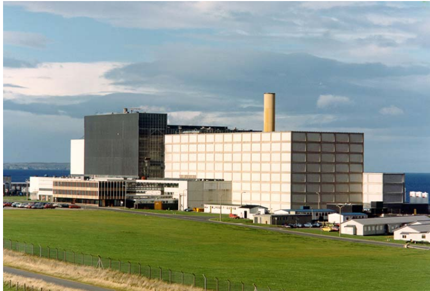
Figure 15: Prototype Fast Reactor (PFR) at Dounreay
