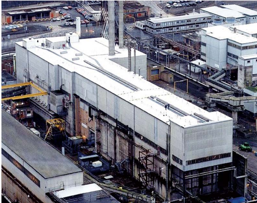
Figure 30: Aerial view of the Magnox Swarf Storage Silo at Sellafield
