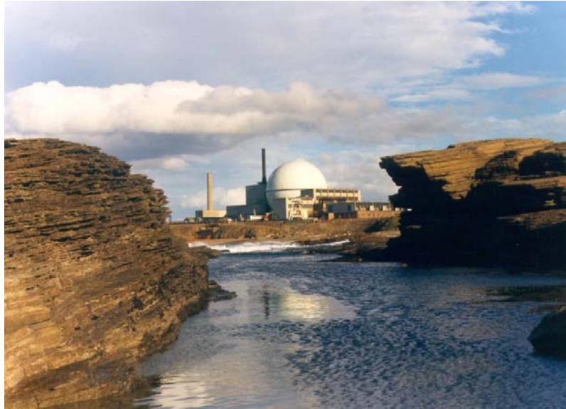
Figure 13: Dounreay Fast Reactor (DFR)
