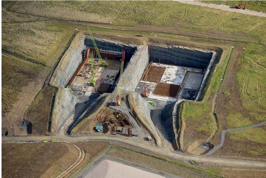
Figure 25: LLW facility whilst under construction at Dounreay
