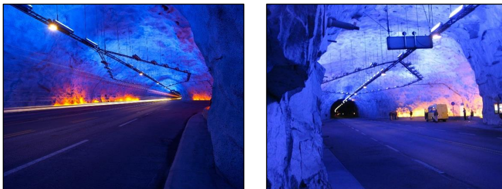
Figure 6-1 – Lærdal Tunnel lighting and cavern
