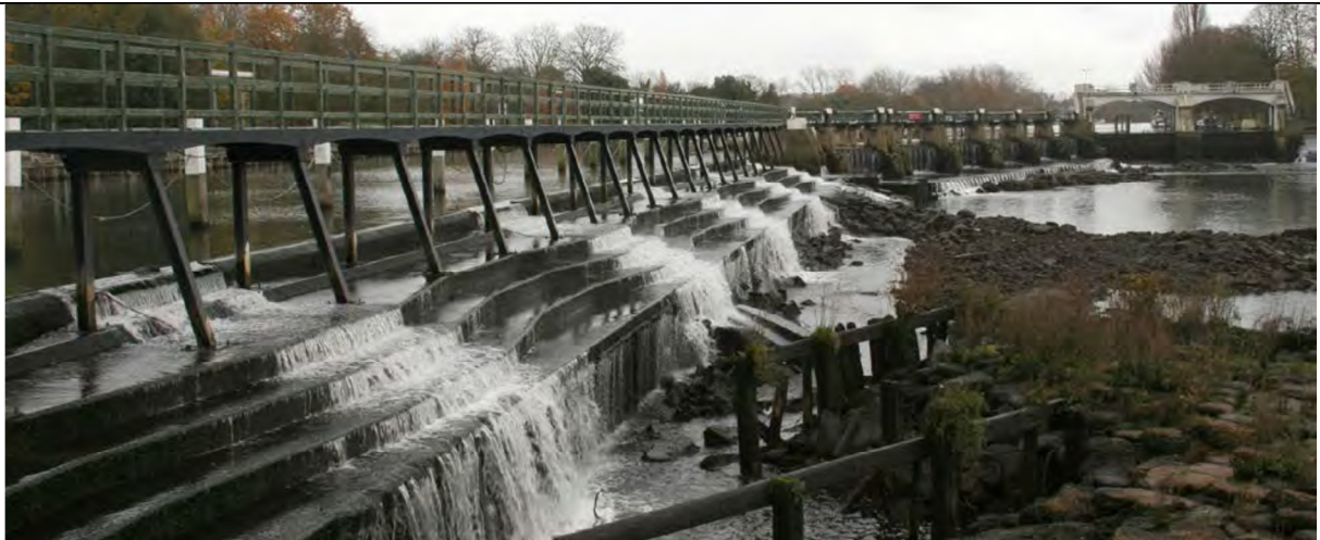
Low winter flow over Teddington Weir – 4 cumecs. 4 December 2011
