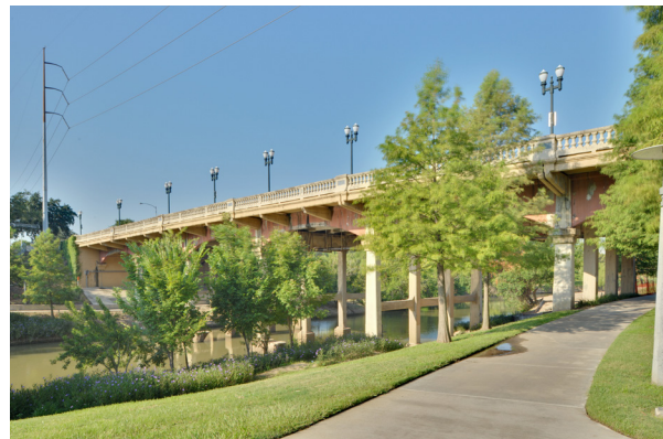
Bridge integrated with adjacent parkland. Buffalo Bayou, Texas ©Ed Uthman
