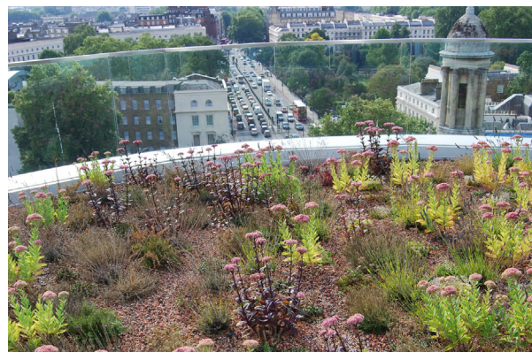
An example of the ecological and aesthetic benefits of green and brown roofs ©Arup
