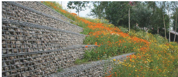
Retaining wall, Queen Elizabeth Olympic Park, London ©Arup
