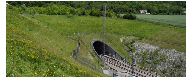
HS1 tunnel portal ©Arup
