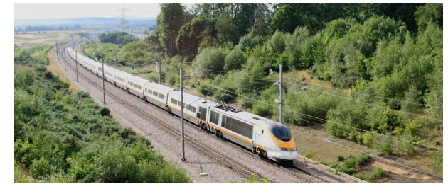
Planting along HS1 provides screening and visual interest ©Arup
