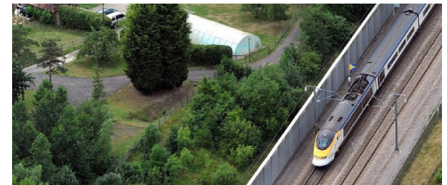
HS1 timber environmental barrier ©Arup
