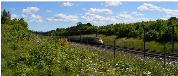
Discreet fence integrated with landscape adjacent to HS1 ©Arup
