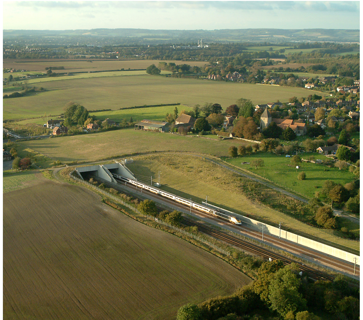
High Speed 1 - Green Tunnel and landscape integration at Mersham, Kent ©Hawk Publications
