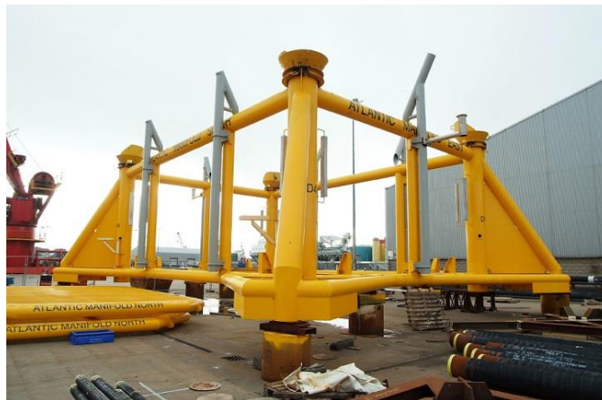
Atlantic Manifold Protection structure (piled at each corner)
