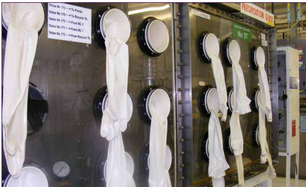
◦ Gloveboxes that formed part of the plant are being taken apart
