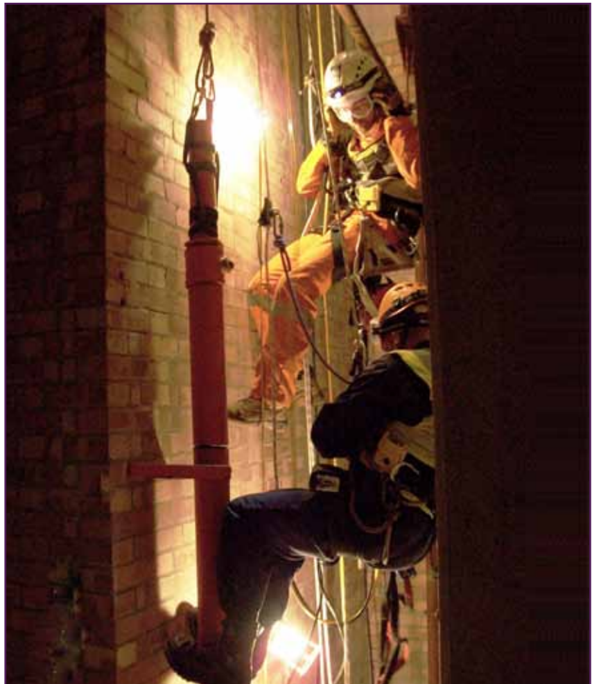
◦ Workmen remove pipework from one of the reactors
