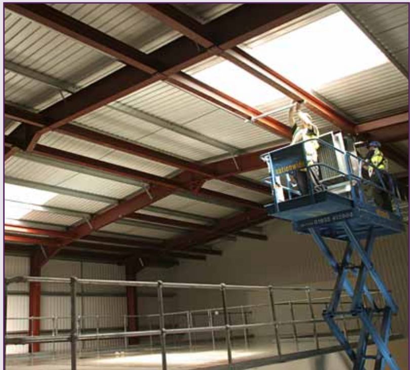
° The Waste Encapsulation Treatment Plant in its early days
