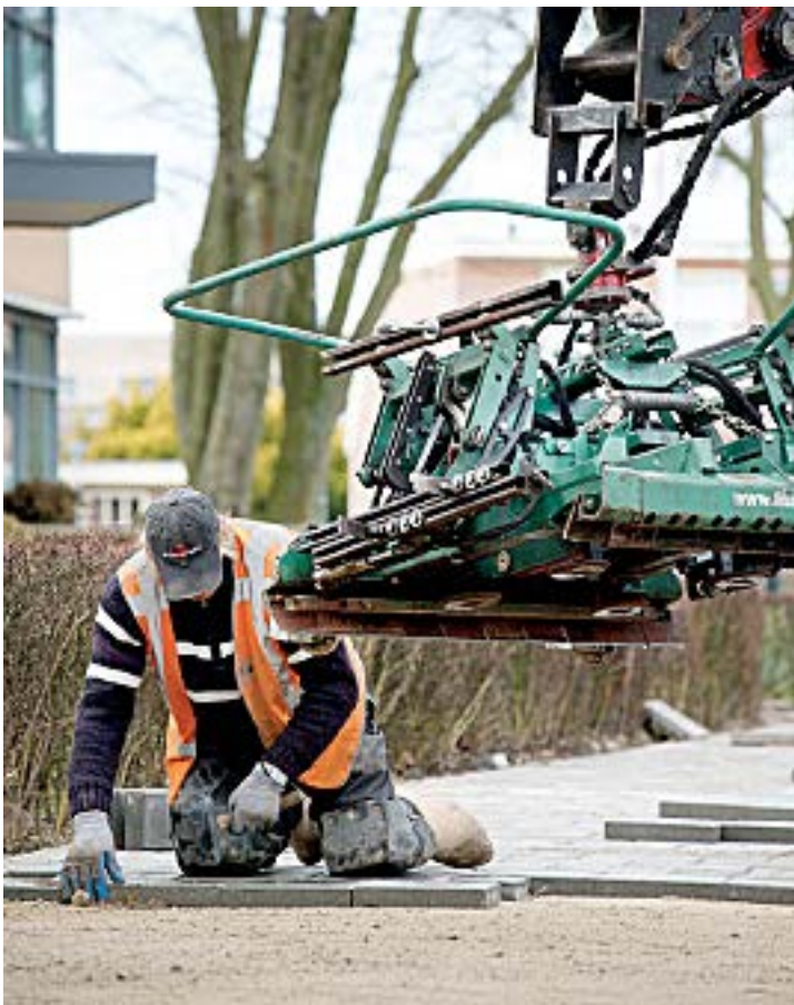
Figure 5: Paving slab handling device (source: TNO, Netherlands)
