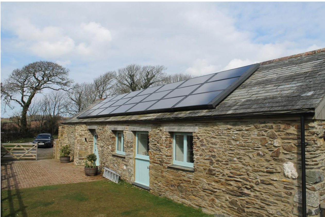
Figure 16 Domestic installation of PV-T. Image courtesy of Anthony Morgan.
