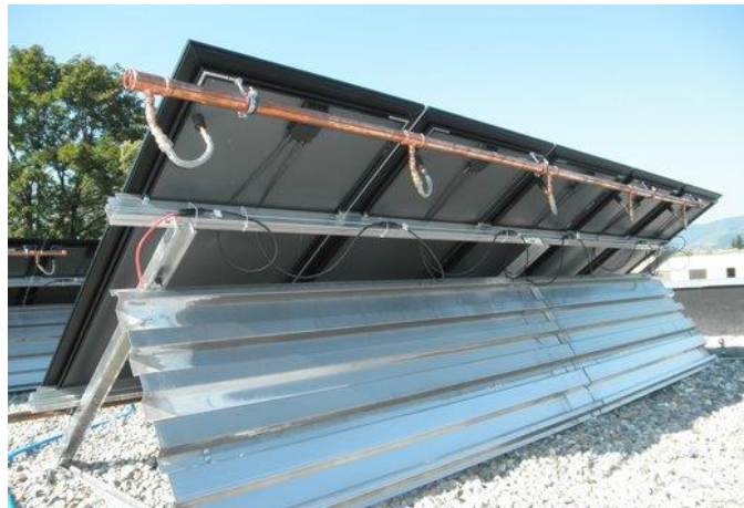
Figure 6 Example of a type 1b unglazed PV-T module, without thermal insulation, heat exchangers as a separate unit under PV module (GSE Air'System and C.Bösch Solator, 2015)
