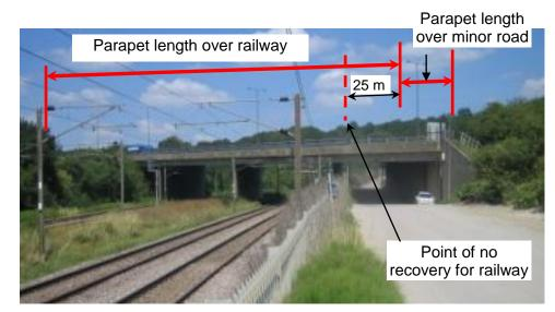
If the lengths in between  $P_{Rail} / P_{Road} / Parapet ends are relatively short, it may be impracticable to have different containment levels from that required at <math>P_{Rail}$  and or  $P_{Road}$ . In
