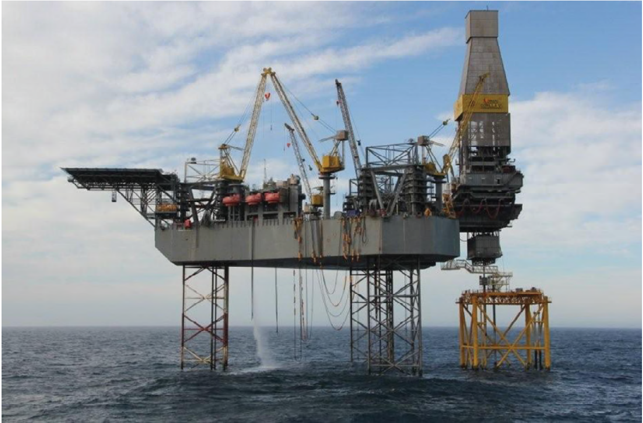
Figure 7 : Drilling Operations CNS
