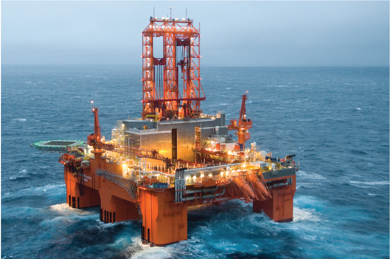
Figure 6 : Drilling Operations WOS
