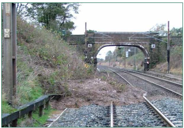
Figure 5: Landslip at Oubeck North looking in the direction of traffic
