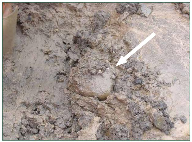
Figure 6: Indication of consistency and boulders in the landslip material
