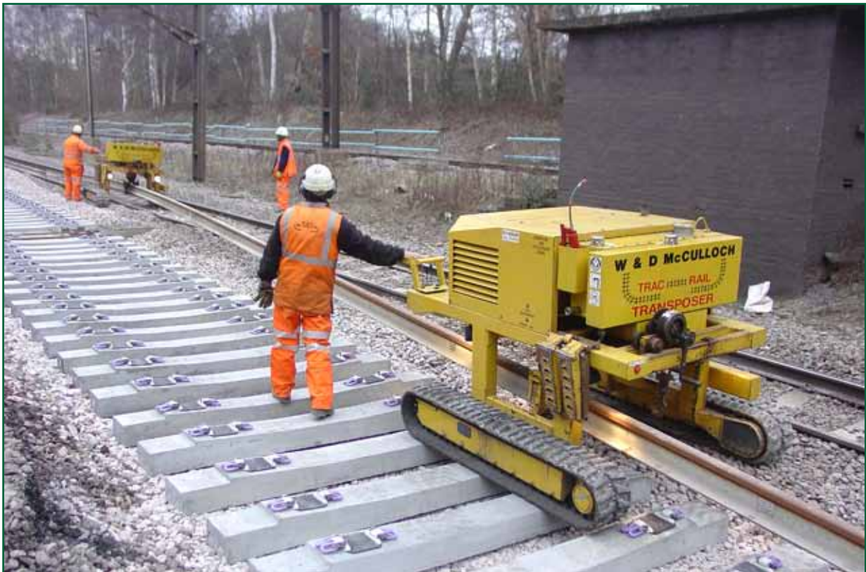
Figure 4: A Trac Rail Transposer in use
