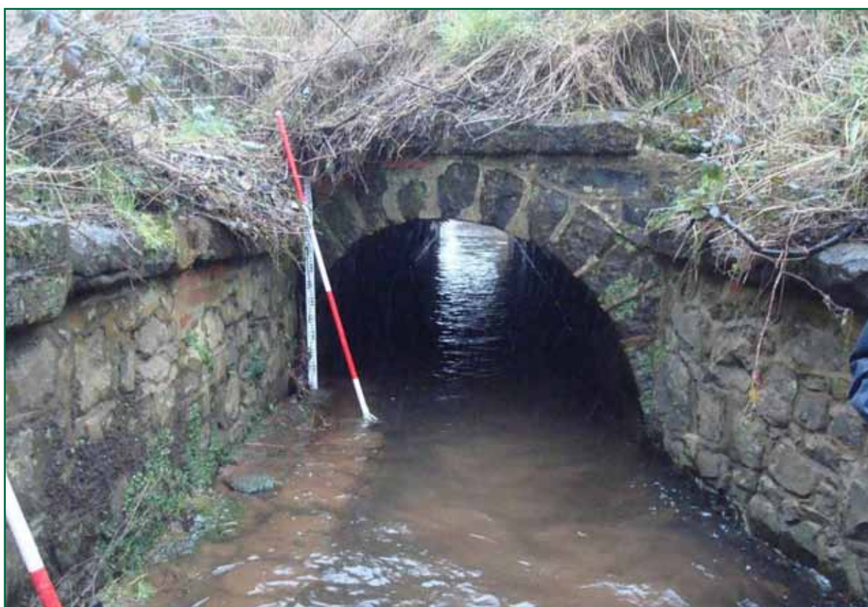
Figure 7: Culvert UB1 inlet under Antrim branch line (image courtesy of URS)
