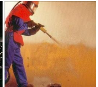
Manual blast cleaning
