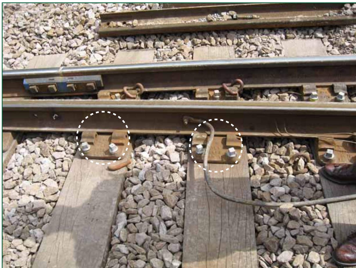
Figure 11: Close up of baseplates with missing fasteners
