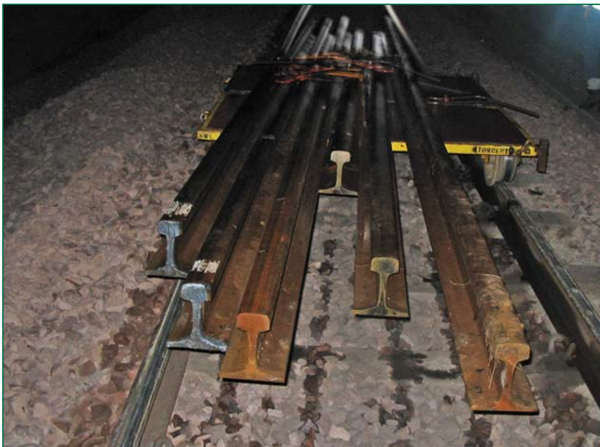
Figure 12: Image taken by the RIO from within Barncluith tunnel
