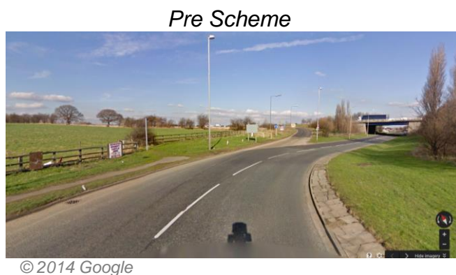
Figure 2-6 M1 Northbound Entry-Slip Road
