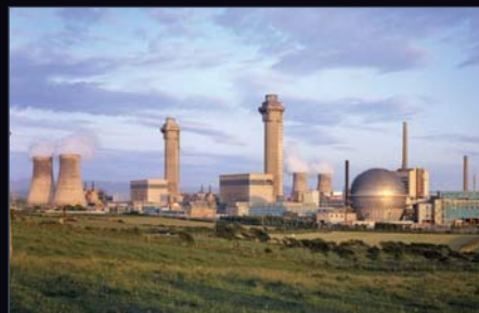
Today, WAGR has served its purpose and has now been safely decommissioned, although the outer sphere remains in place
