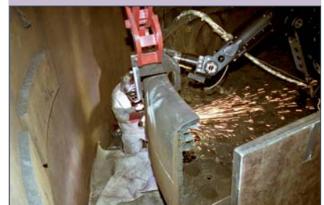
More work to dismantle the reactor core and pressure vessel
