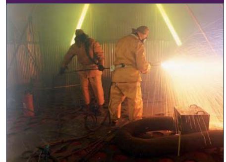
Cutting the Top Biological Shield
