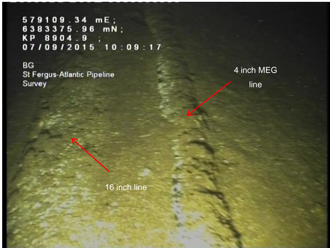
Figure 13 – Typical “Type A” surface-laid pipeline showing partial burial (2015 survey)
