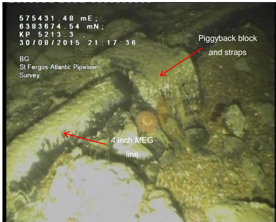
Figure 20 – “Type C” rock-covered pipeline showing minor exposure (2015 survey)
