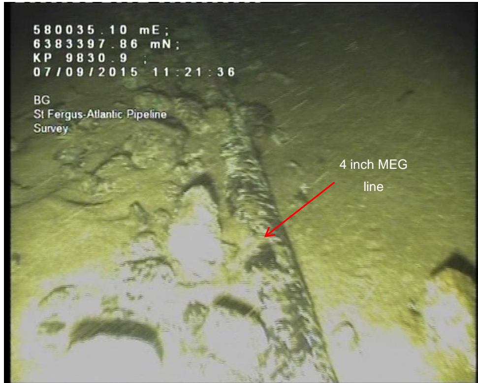
Figure 17 – Typical “Type B” rock-covered pipeline showing minor exposure (2015 survey)
