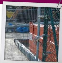
Secured fuel tank in secondary containment
