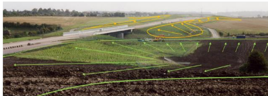
An HS1 railway crossing with arrows highlighting landscape earthworks ©Arup
