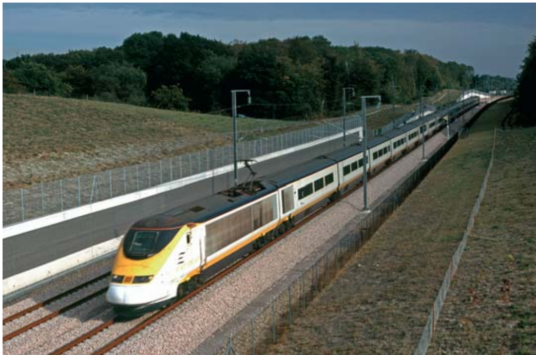
A Eurostar travelling on High Speed One, alongside sound insulating walls and embankments
