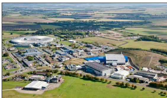
Aerial photo of Harwell Oxford campus
