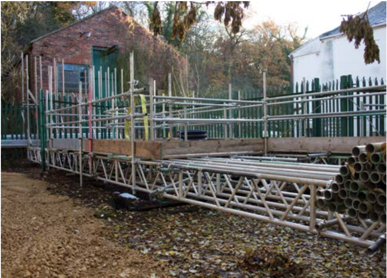
Mine entry repair work in the North East
