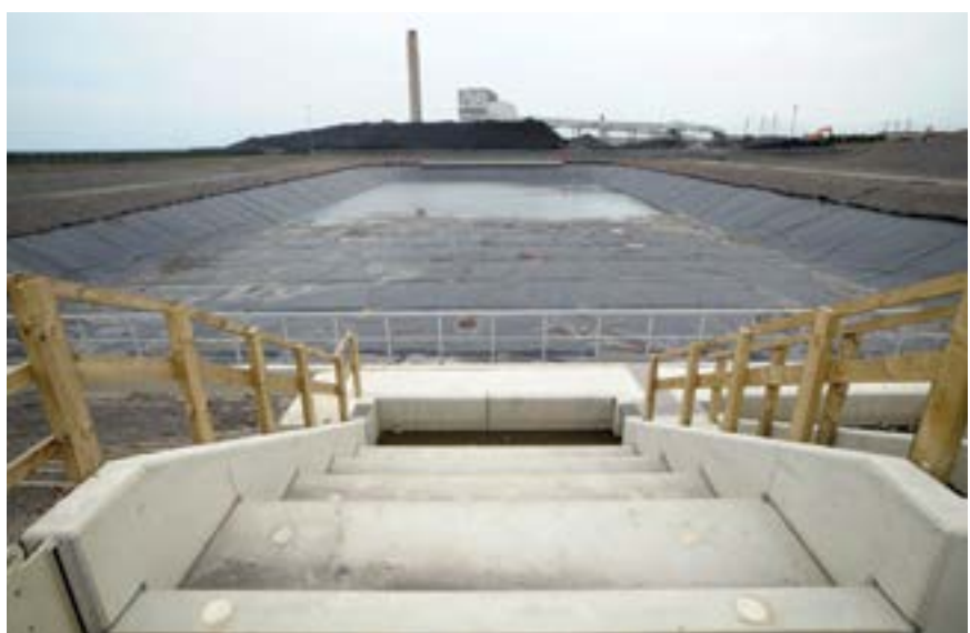
Construction of Ellington mine water treatment scheme
