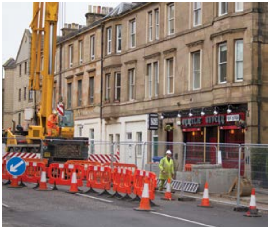
Public safety and subsidence work at Joppa, Scotland
