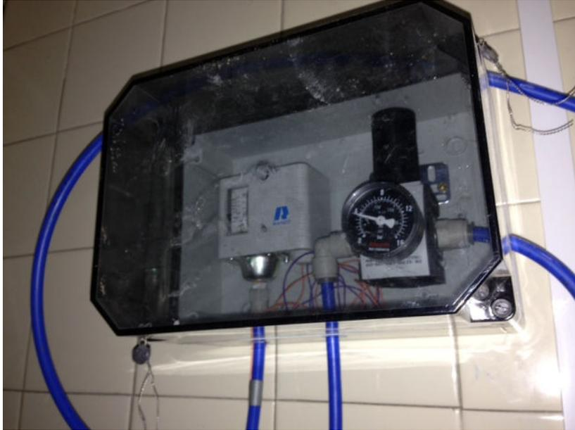
**Figure 9** Pressure sense switch and regulator housed in a single clear case
