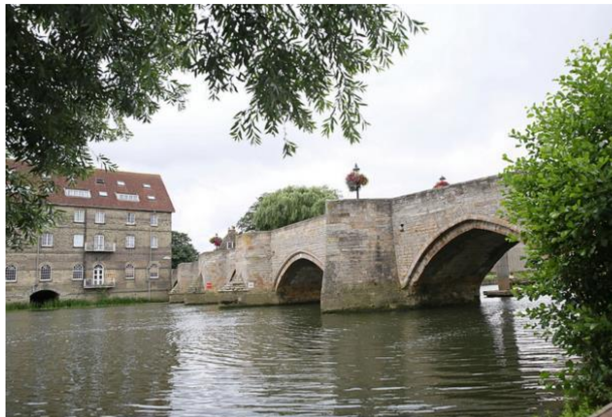
Plate 6.1: The medieval Huntingdon Bridge
