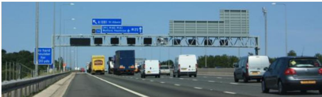
Figure 5-15– Superspan gantry on the anti-clockwise carriageway approaching Junction 22
