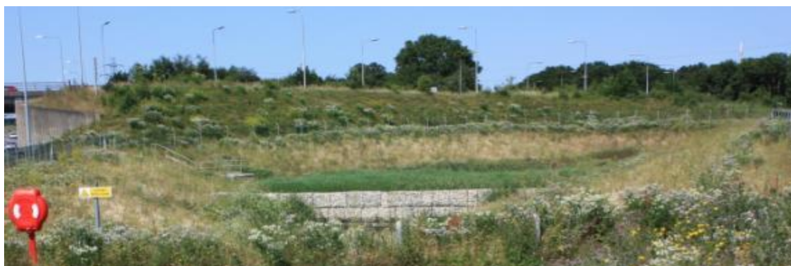
Figure 5-25– Pond 27a at Junction 22
