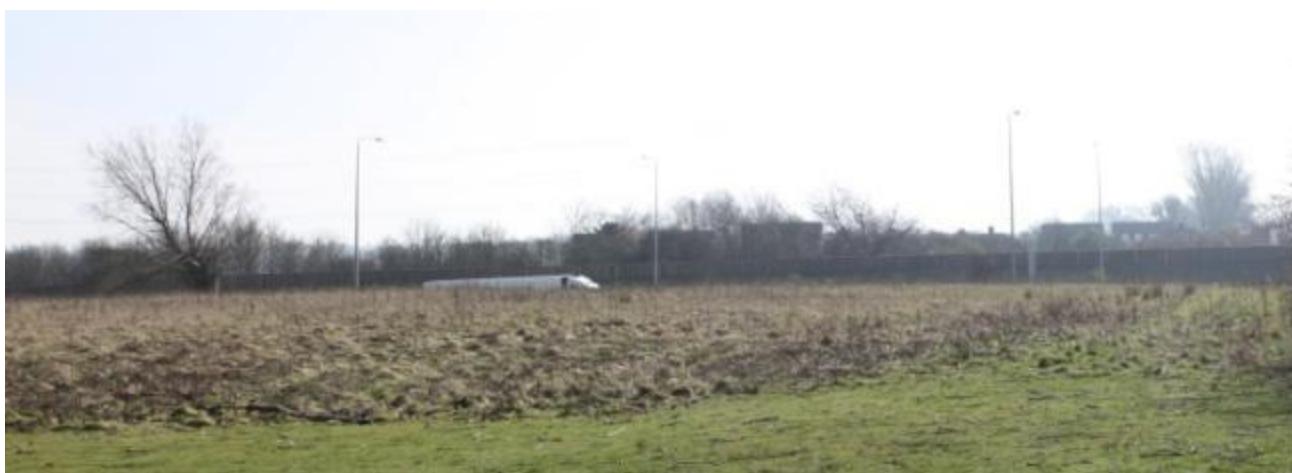
One year after scheme opening – photograph taken in March 2014
