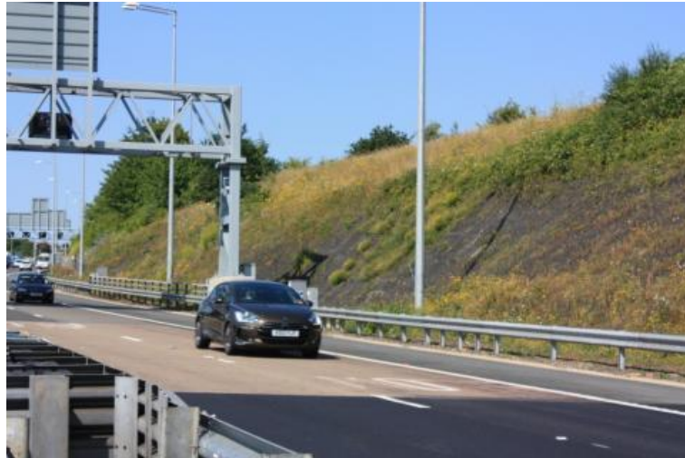
Figure 5-1– Matting on steep chalk slopes near junctions 17 and 18
