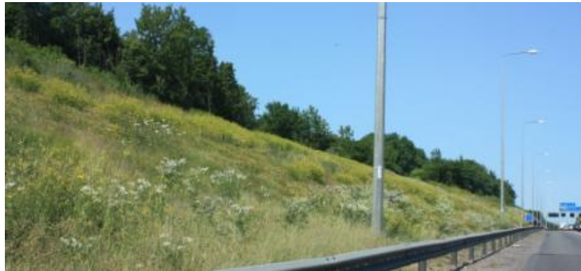
Figure 5-10– Slope demonstrating seeding success as well as occupation by the seed source contained within the topsoil
