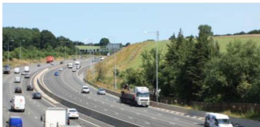
Figure 5-7– Land purchase slope visible on the right-hand side (anticlockwise near junction 18) – re-grading replaces sheetpile feature
