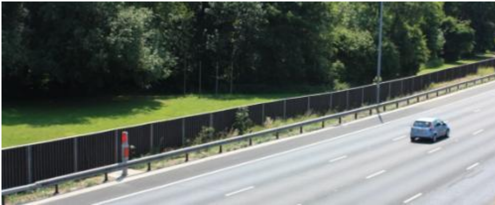
Figure 5-4– New Environmental Barrier located on the approach to Junction 18 off slip (anticlockwise)
