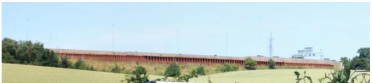
Figure 5-6– Sheetpile retaining wall and noise barrier near junction 17
