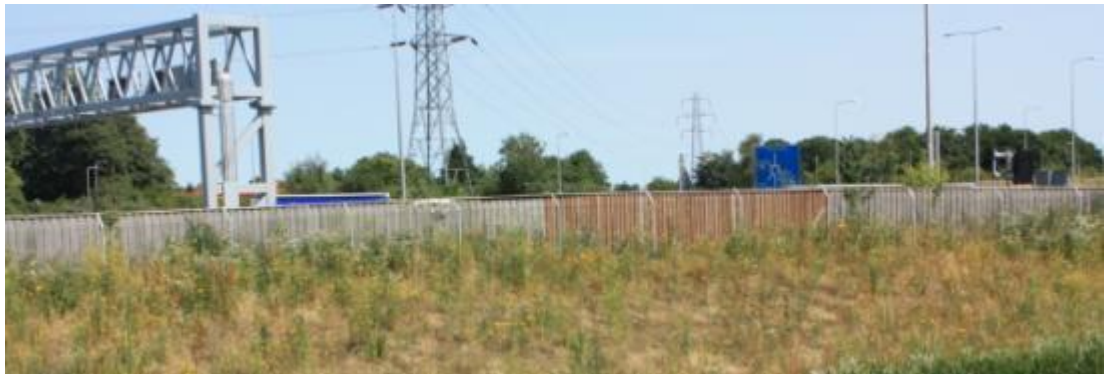
Figure 5-16– New gantries, environmental barriers, signs and lighting add to the increased visual intrusion of the scheme
