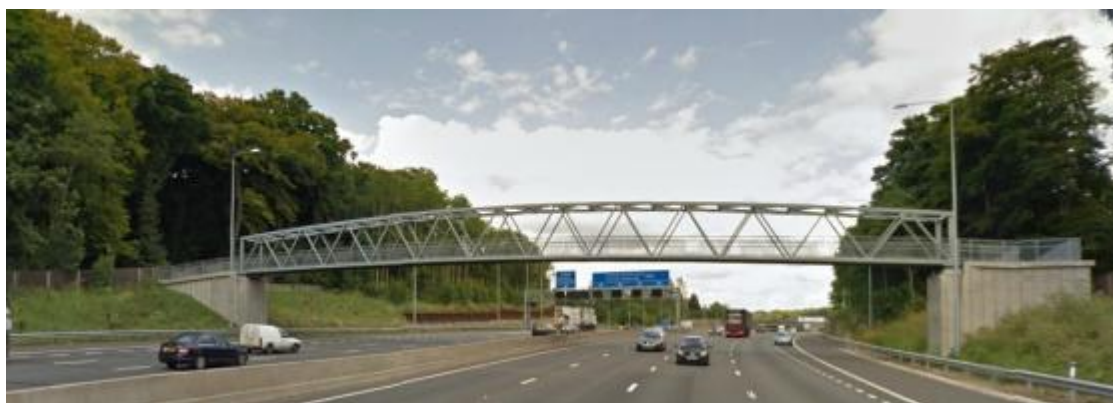
Figure 5-26– Park Lane footbridge near junction 18 – new structure replaced original bridge
