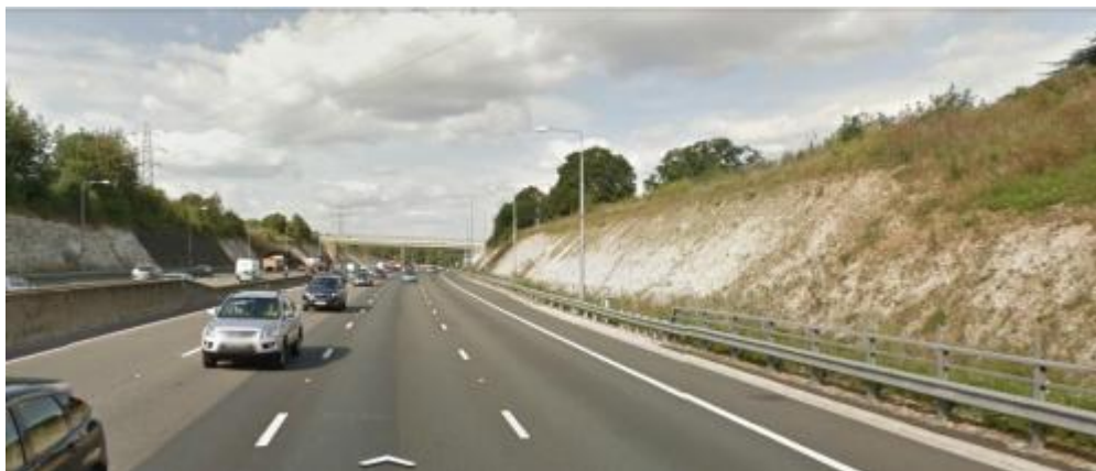
Figure 5-17– Reduced height light columns and overhead cables near Hornhill Lane (image from Google Maps)
