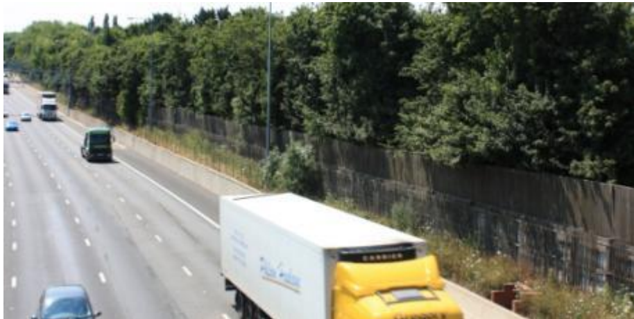
Figure 5-3– Retained Environmental Barrier near Junction 18 (clockwise)
