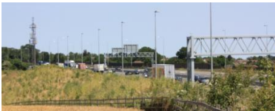
Figure 5-14– Chorleywood bund near junction 17 – planting on bund will ensure increased screening of the motorway, in addition to that achieved by the bund earthworks
