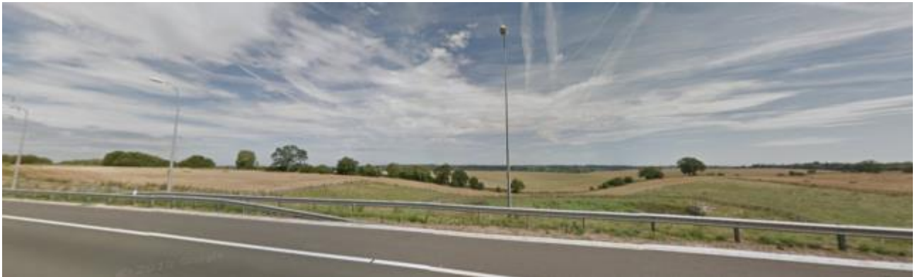
Figure 5-18– Reduced height light columns and overhead cables near Shenley Lane (image from Google Maps)
