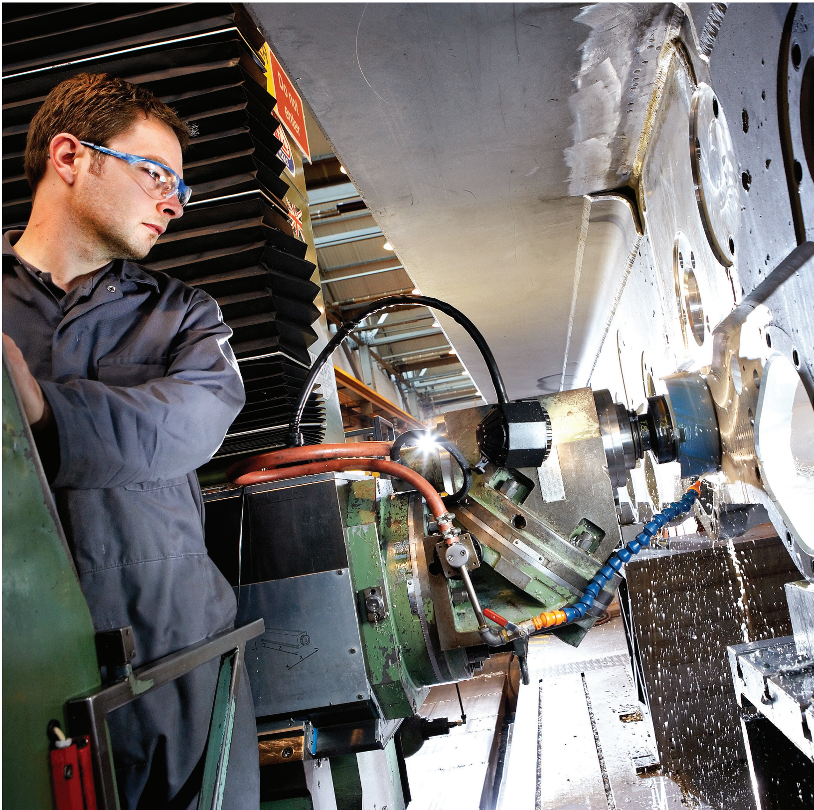
Above: Donnington team member repairing a Warrior hull using the Elgar mill.
