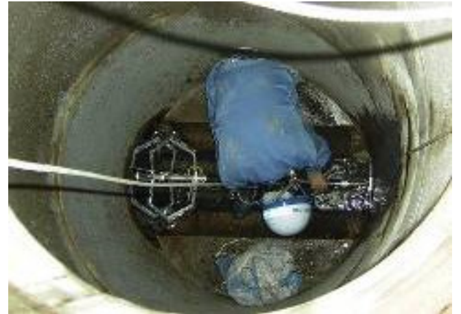
Figure 3 - Inertial gyroscopic device being inserted into pipe
